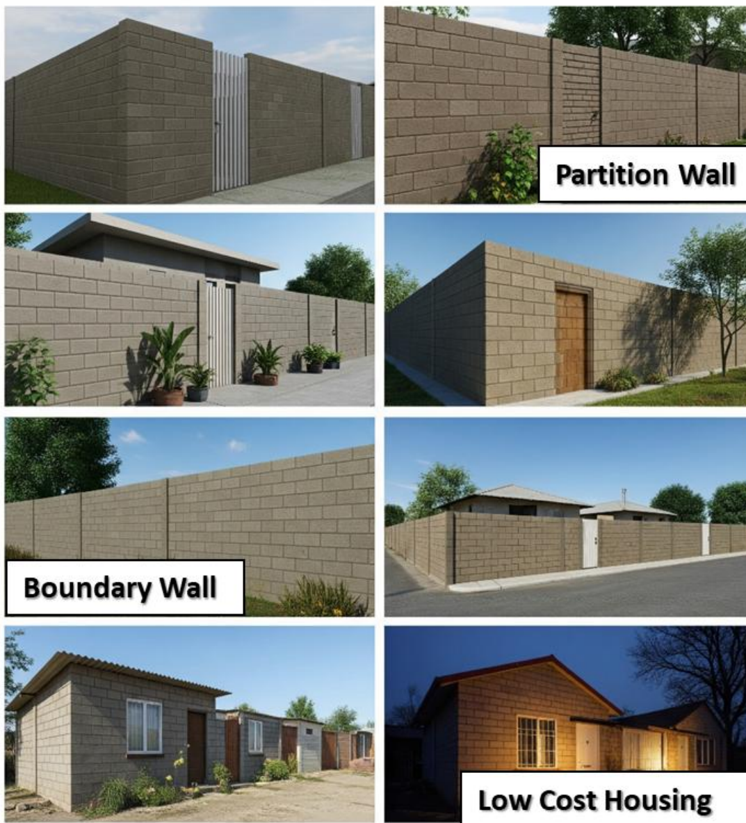
Figure 1: Use of fly ash-clay bricks in non-load bearing wall including partition wall, boundary wall and low cost housing
